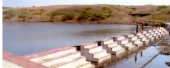
After the monsoons, a survey of improvement in ground water level was carried out. The data collected for various open wells and tube wells directly affected by Anicut shows an average rise of 13.73 ft in water level of open wells and 112 feet in case of tube wells. Looking at the persistent drought conditions over last three years, this rise in water level is encouraging.
